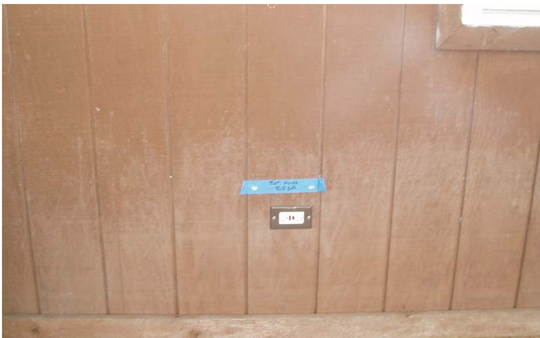
Fig. 25b– House IL-5, Non-Operational GFCI Receptacle With No Outdoor Faceplate or Box Cover (closer view of Fig. 25a)
