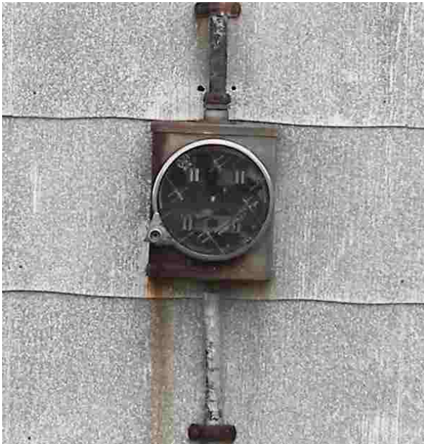
Fig. 10 – Meter Socket With Corrosion From House NY-1
