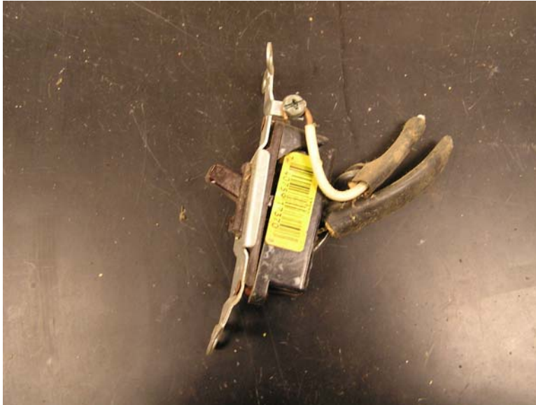
Fig. 32 – House TX-1, White Colored Grounding Conductor
