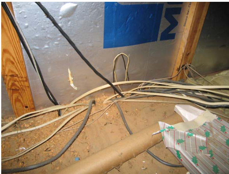
Fig. 39 – House VA-1, NM Cable Not Supported by Staples
