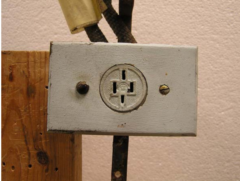
Fig. 19 – House IL-6 Receptacle From the Early 20 th Century
