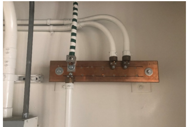
Photo courtesy of J. Montross Ground Bus with grounding connections
