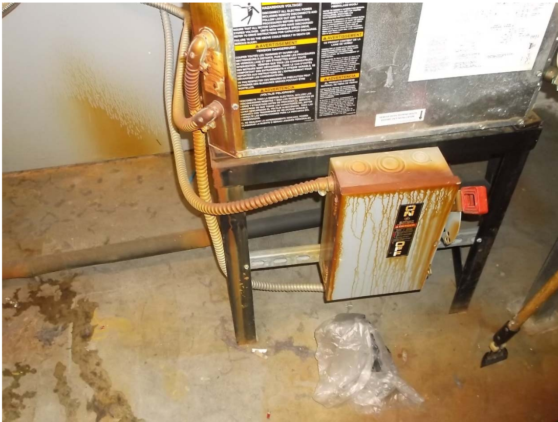
Figure (H4c): Another view of rust stains caused by pinhole leaks.
