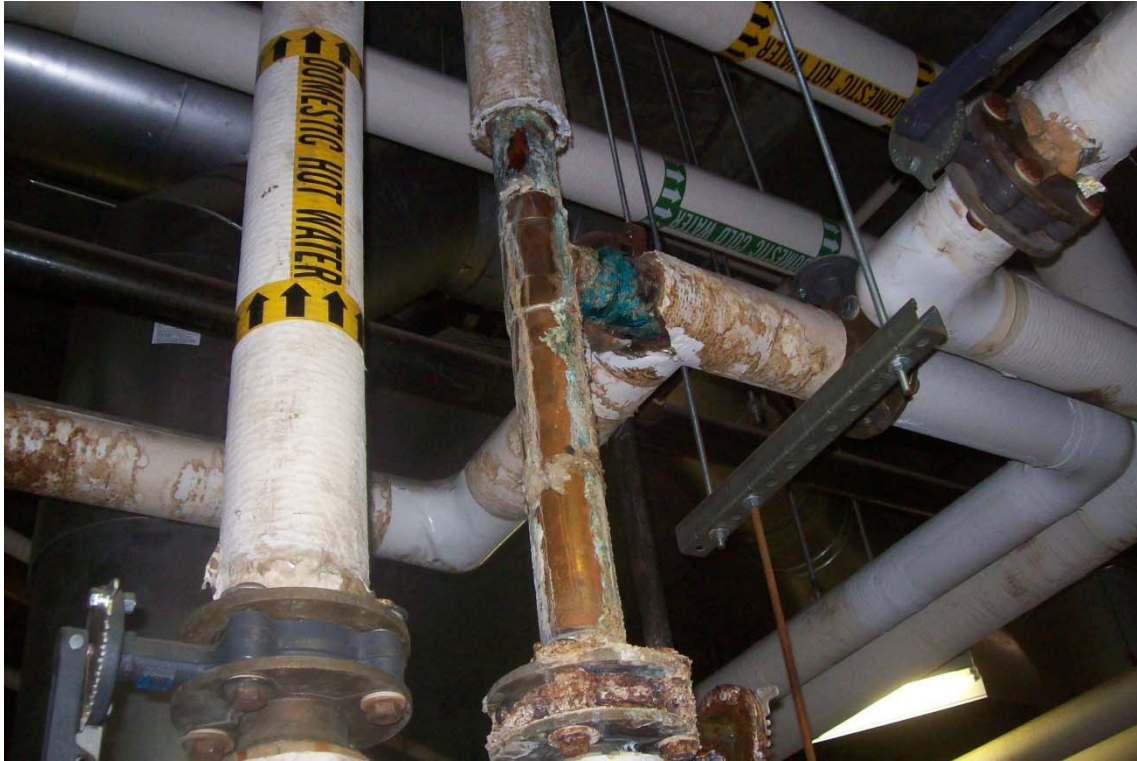
Figure (H1d): A view of typical piping corrosion where the solder joints had failed.
