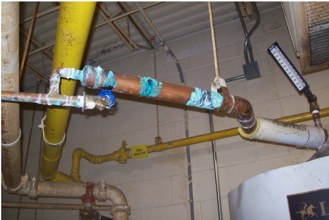
Figure (H3b): A view of pinhole leaks within a mechanical room.
