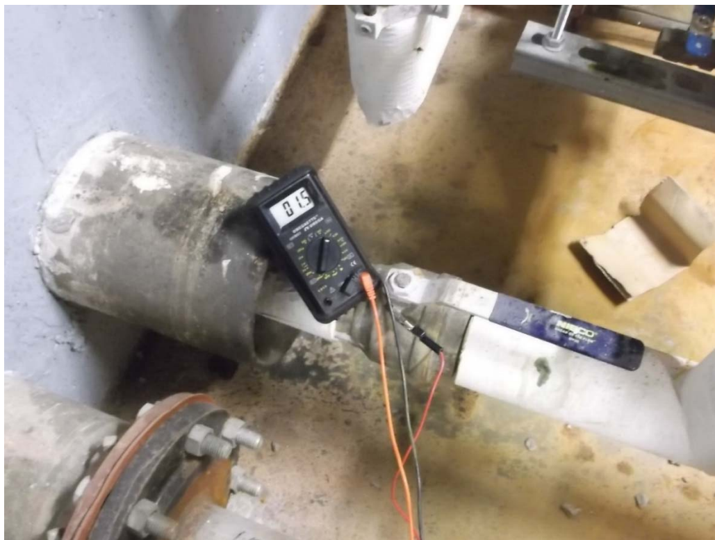
Figure (H4e): A view of 15 mA of DC flowing on the domestic water piping (pipe to building steel). Later that day we observed 20 mA.
