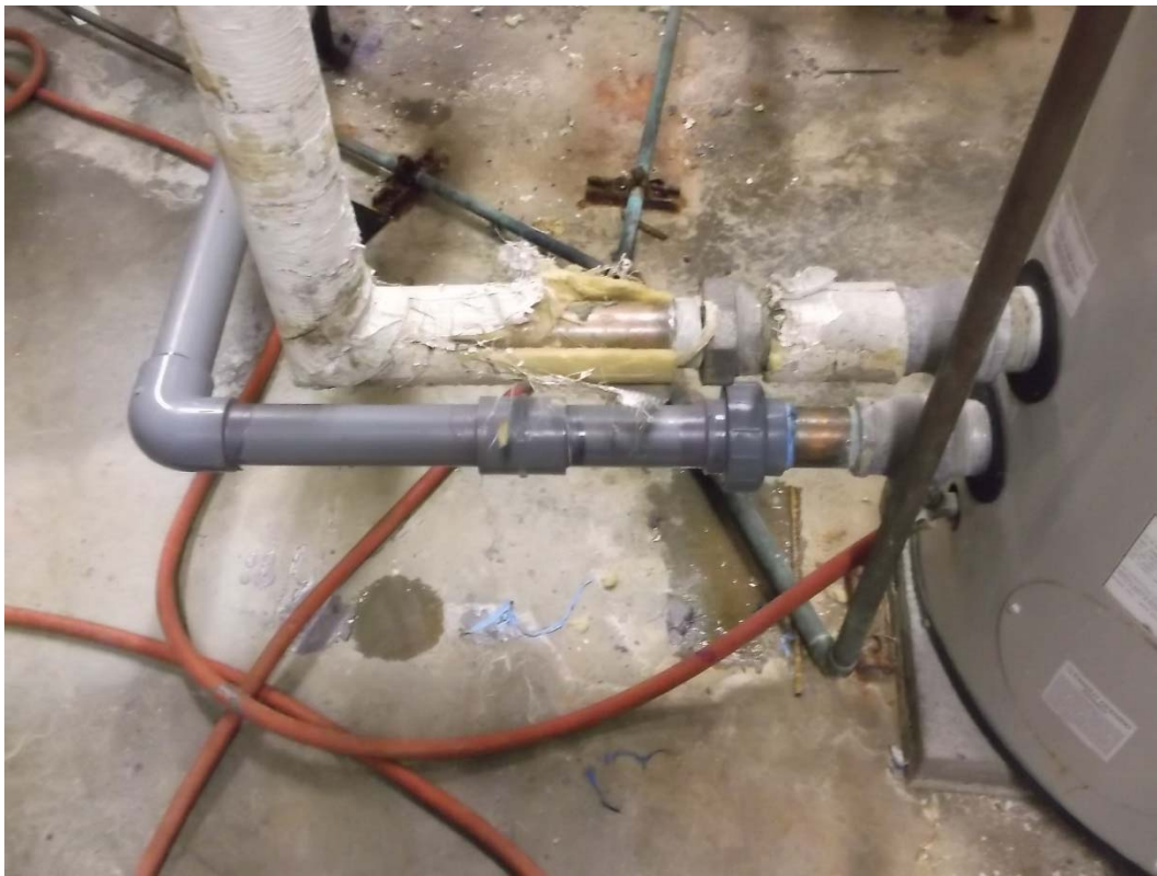
Figure (H3d): A view of failed copper piping removed and replaced with CPVC (plastic piping). Ultimately, the entire facility was repiped with CPVC (domestic hot and cold water piping).
