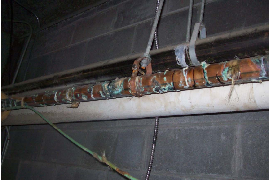
Figure (H3a): A view of pinhole piping failures that were typical throughout the facility.
