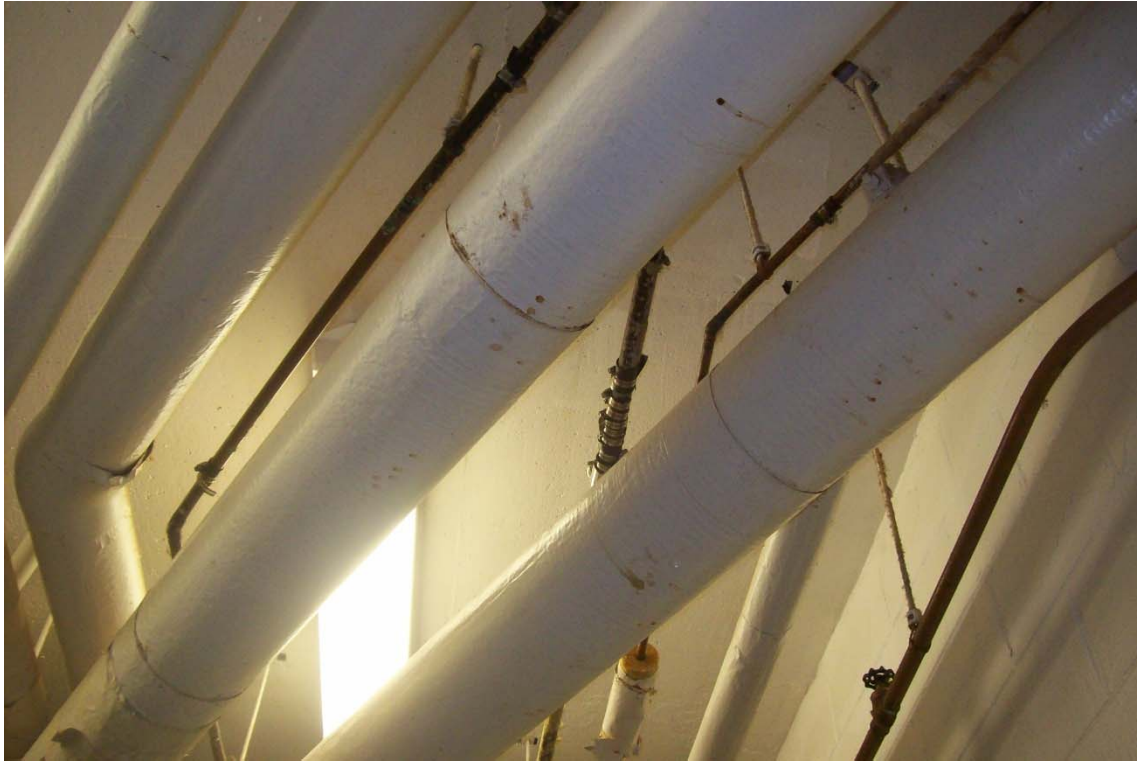
Figure (H2b): A closer view of typical pinhole leaks. At each pinhole leak, a rubber strip with hose clamp is applied, as a temporary repair.
