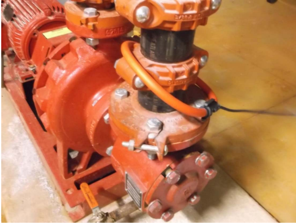
Figure (T1b): A view of the inductive donut sensor used on the HVAC piping (at the HVAC loop pump).
