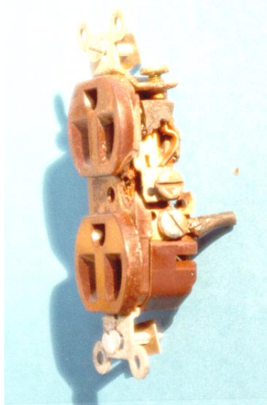
Figure 1 - A Receptacle Damaged by a Glowing Connection
