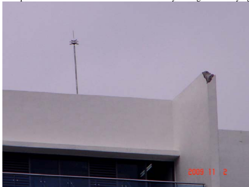
Above: The Serai Saujana Condominium which was installed with the PDC air terminal. Below: A close-up view of the PDC air terminal and the nearby damage caused by lightning.
